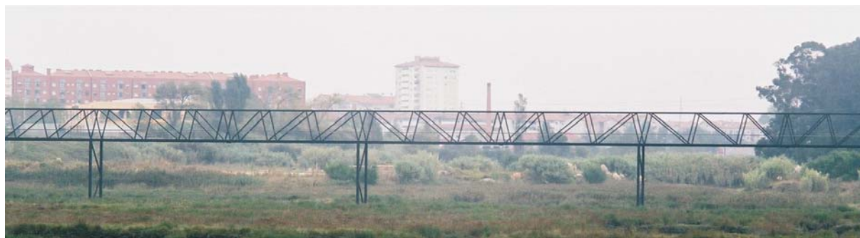
Figura 6. Ponte pedonal – vista lateral.
