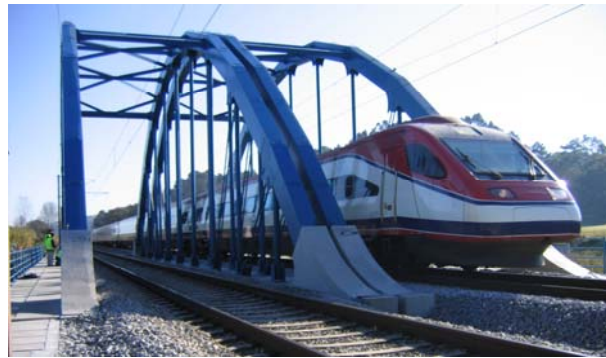
Figure 3. São Lourenço bridge
